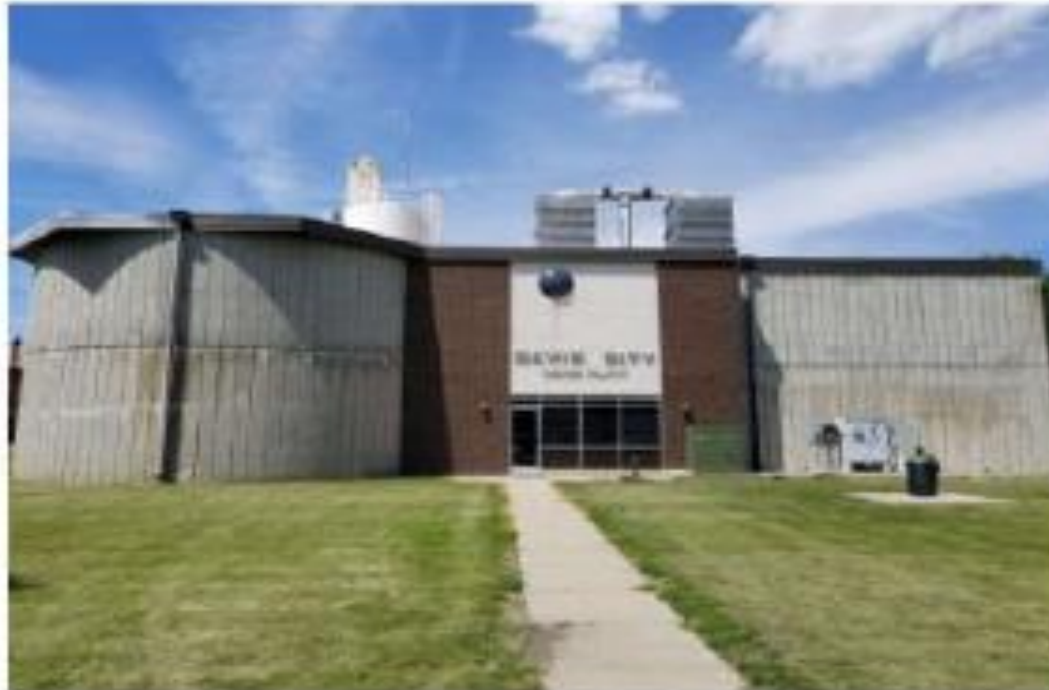
Figure 8. David City WTP
