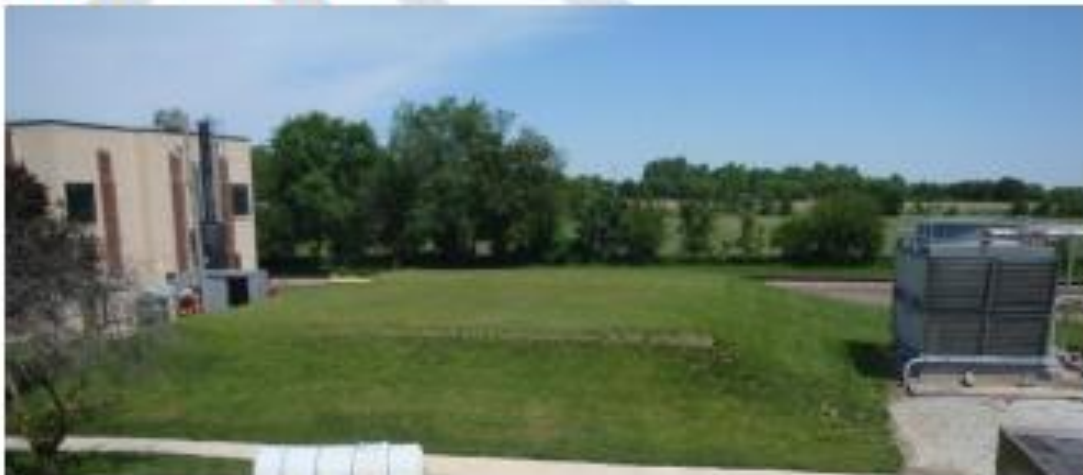
Figure 7. WTP Clearwell Site
