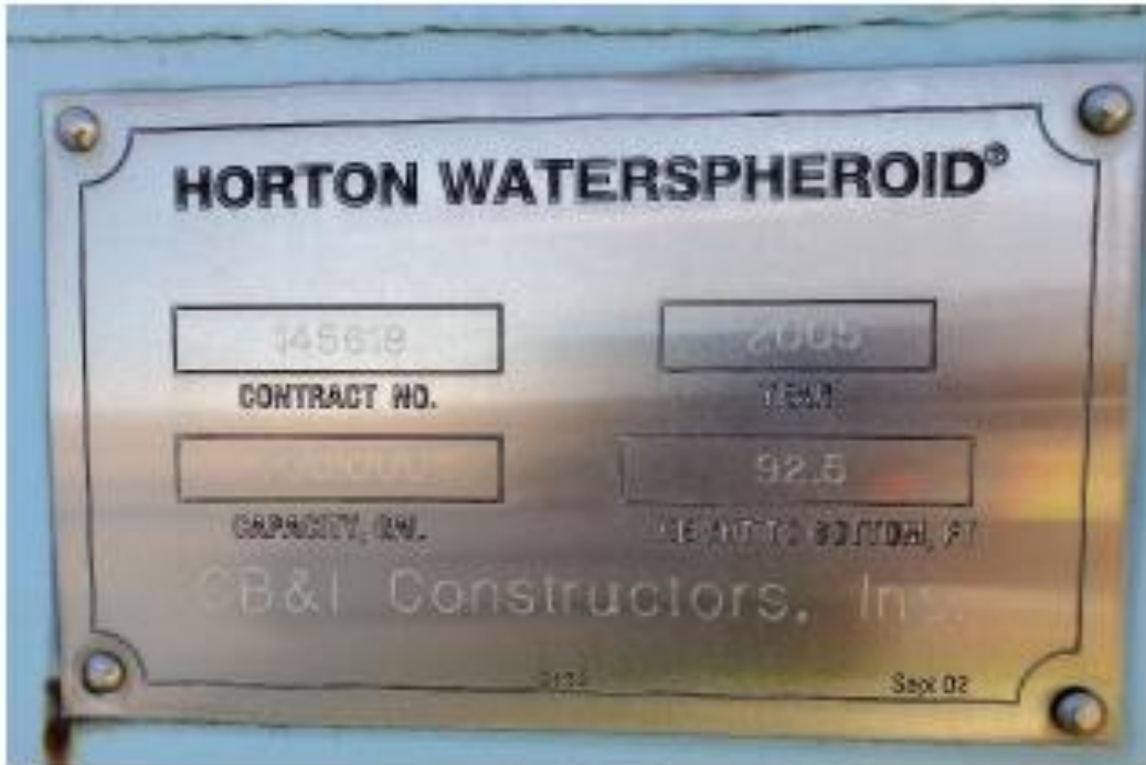
Figure 6. 750,000-gallon Tank Nameplate
